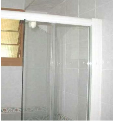
Framed; the fixed panel
