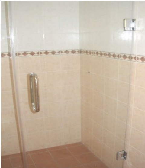
Frameless; swing door fixed to wall to fixed panel
