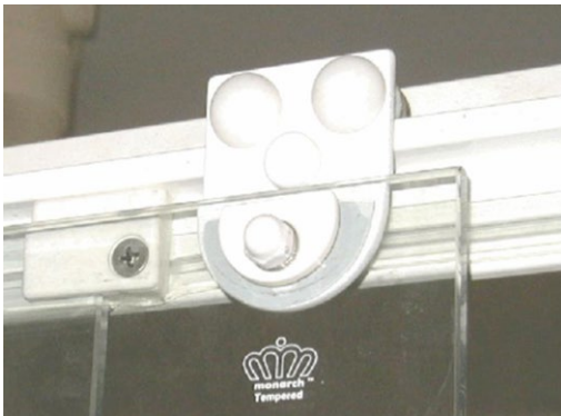
hanging rollers and/or sliding guide; has dislodged, damaged or missing.
