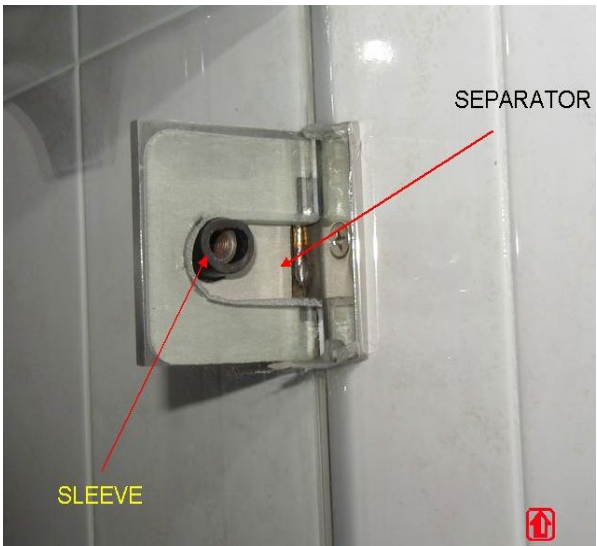
separator between glass and metal parts; missing or out of position.
