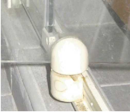
Pivot hinges; has cracked or dislodged.
