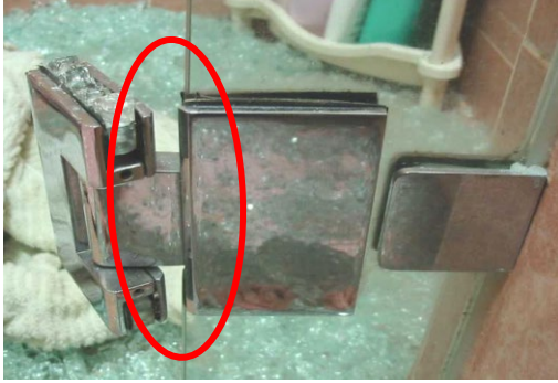
door hinges; the pair were not in alignment with each other.
