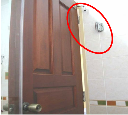
door stopper, flipper weather strip; are missing, damaged or dislodged
