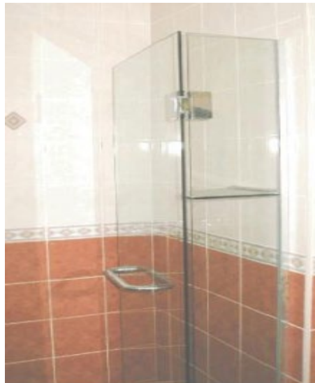
Frameless; swing door fixed to wall to fixed panel
