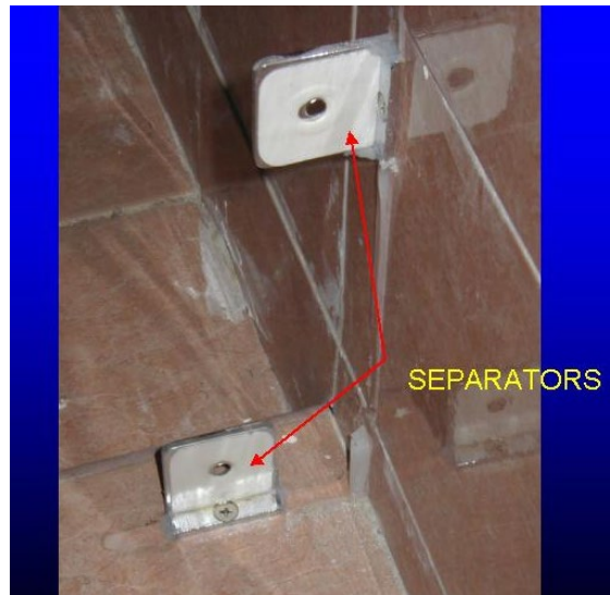
separator between glass and metal parts; missing or out of position.
