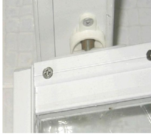
Pivot hinges; has cracked or dislodged.
