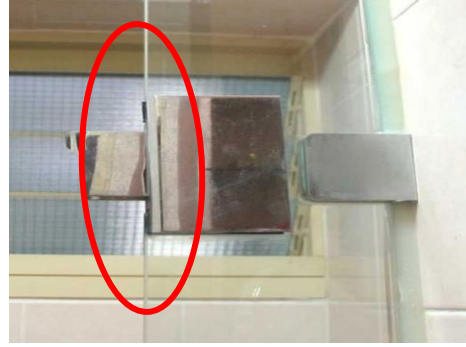
door hinges; the pair were not in alignment with each other.
