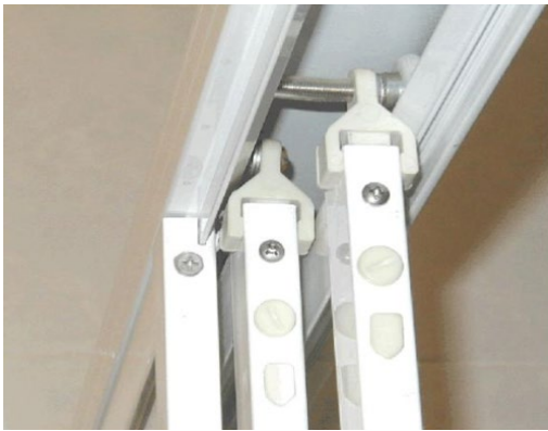
hanging rollers and/or sliding guide; has dislodged, damaged or missing.
