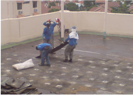
1. Removing existing membrane
