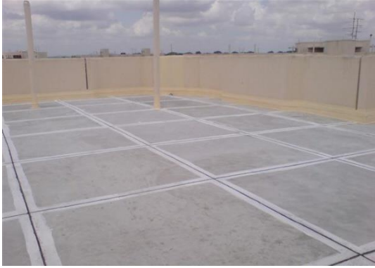
7. Completion of concealed waterproofing system
