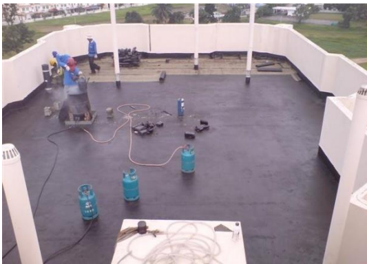
3. Laying of waterproofing membrane
