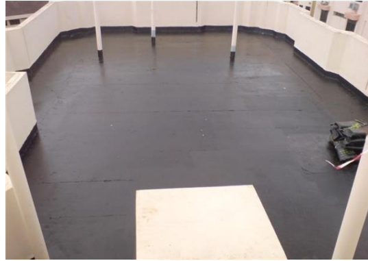
2. Primer has been applied on roof
