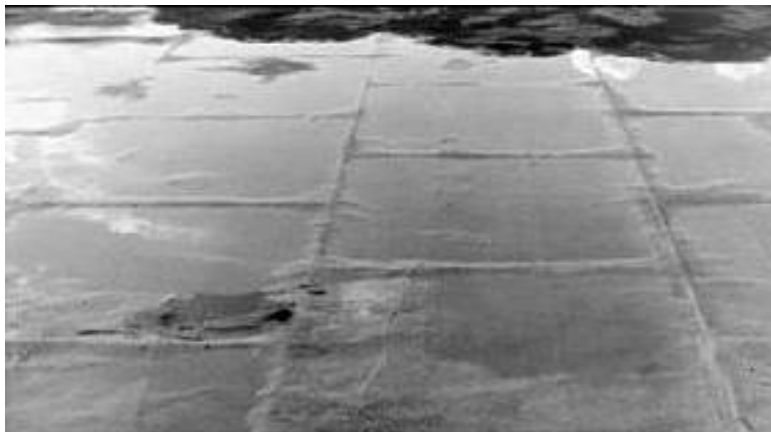
Figure 3 The staggered grid pattern is called picture framing (Griffin & Fricklas, 2006)
