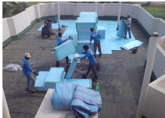
4. Laying of insulation foam over new waterproofing membrane
