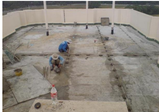
6. Laying cast-in-situ cement sand panel over
