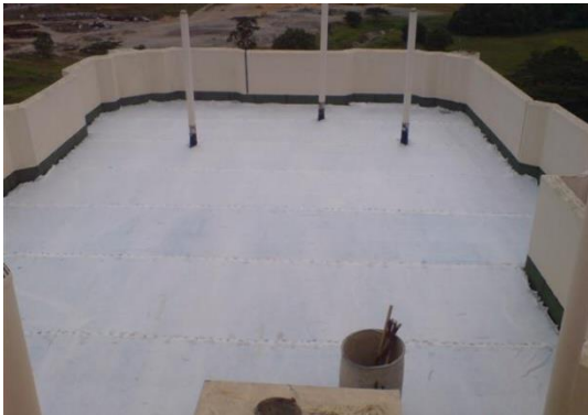
5. Laying of separating geotextile over the insulation foam
