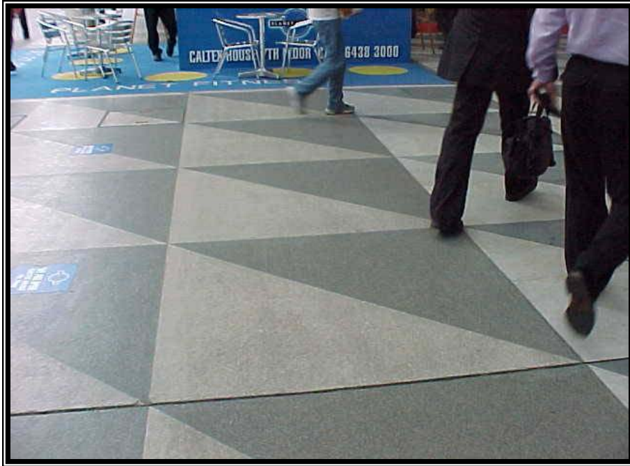
Photo 8 – Close-up view of the epoxy floor system
