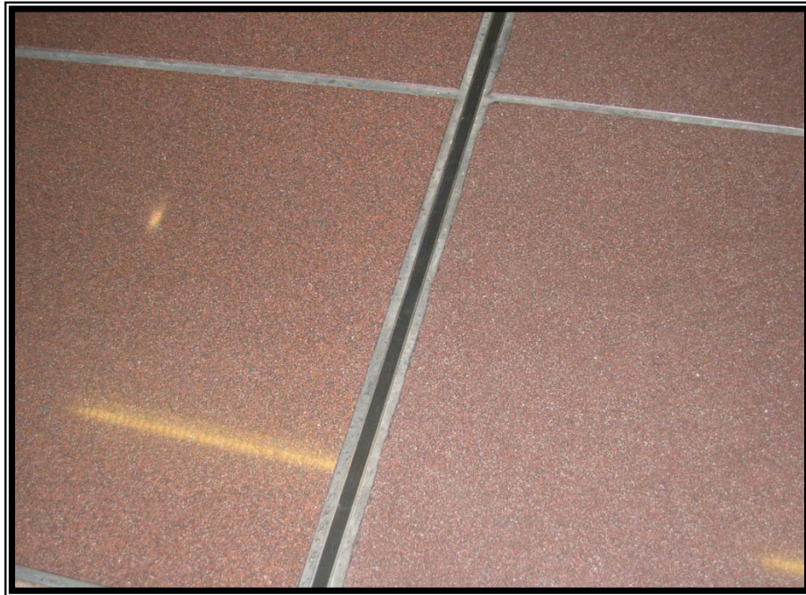
Photo 5 - Existing expansion joints provided on site
