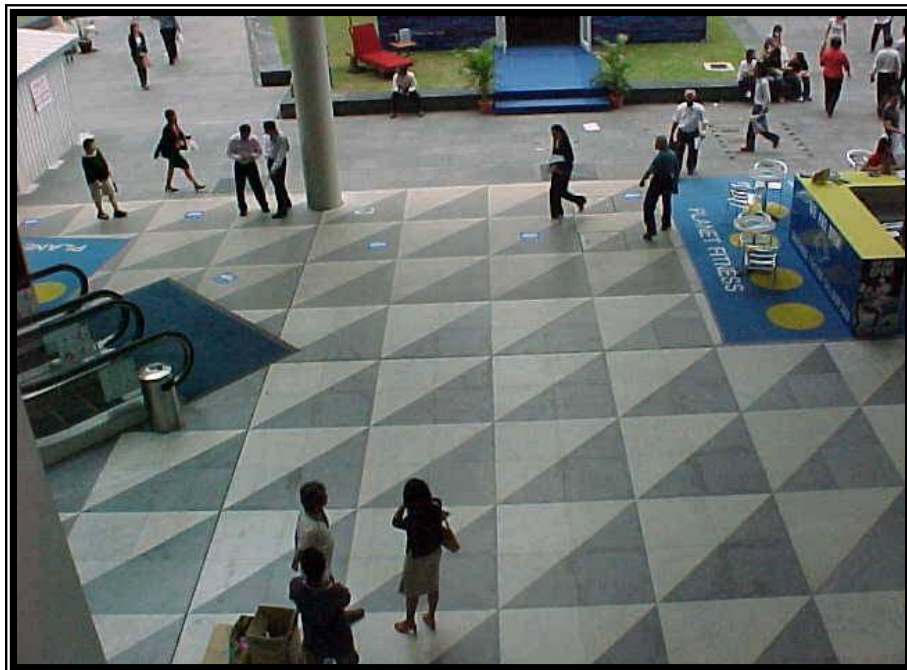
Photo 7 – Epoxy floor coating at Shell Tower
