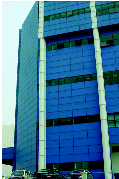
Figure 3.32. Aluminum panels can be fabricated in many colours.
