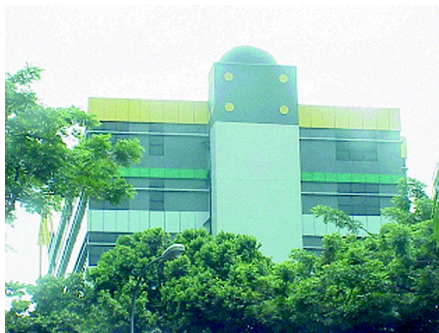
Figure 3.32. Aluminum panels can be fabricated in many colours.
