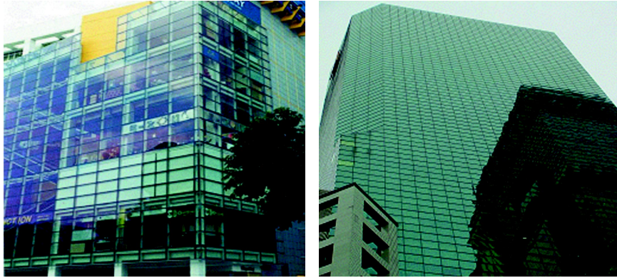
Figure 3.42. Glazed facade with different tints and reflectivity.
