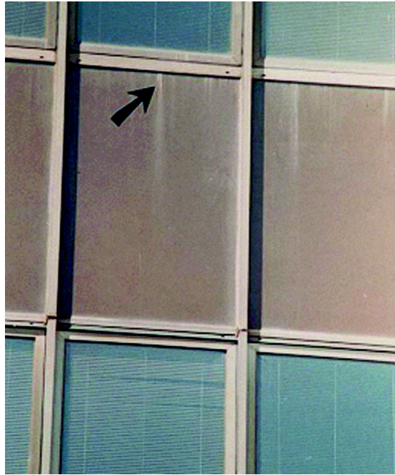
Figure 3.35. Staining on enamel steel
