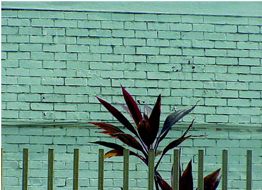
Figure 5.2. Painted brick wall.
