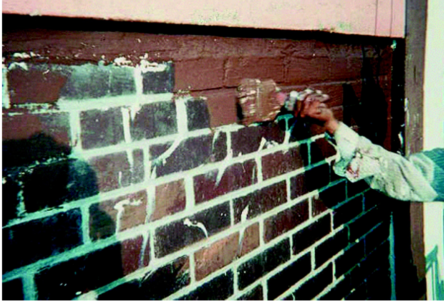
Figure 5.1. Painting over a brick wall.
