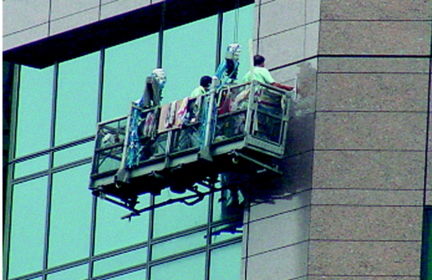
Figure 5.3. Cleaning of facade consisting of glass and natural stone.
