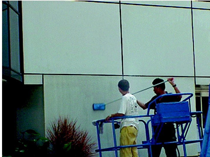
Figure 5.4. Cleaning aluminum panels with a scrub.
