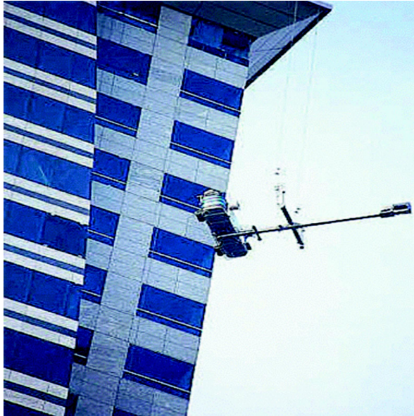
Figure 5.6. A specially designed gondola to reach inaccessible areas.
