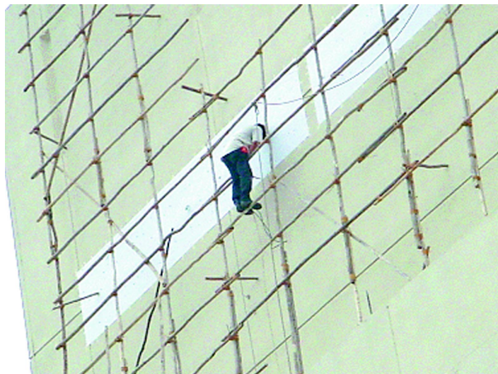
Figure 5.23. Bintagor scaffolding is very popular among developing countries due to its low cost and sturdy framing members.
