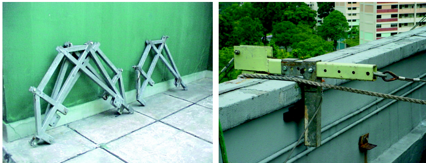
Figure 5.21. Parapet clamp as used on a parapet wall.
