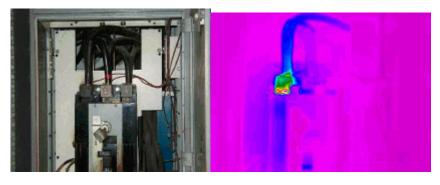
By measuring the temperature profiles of the equipment, infrared imaging produces thermal maps that reveal electrical problems that otherwise would be undetectable.
