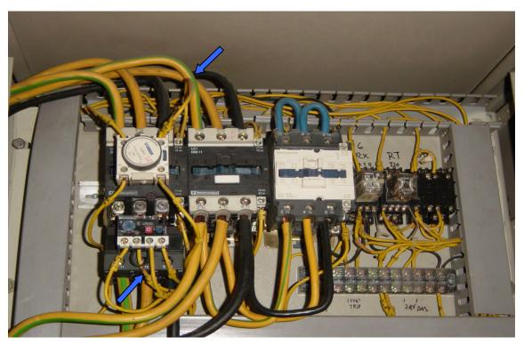
Improper cable terminations are dangerous and may lead to discharge and eventually flash over.
