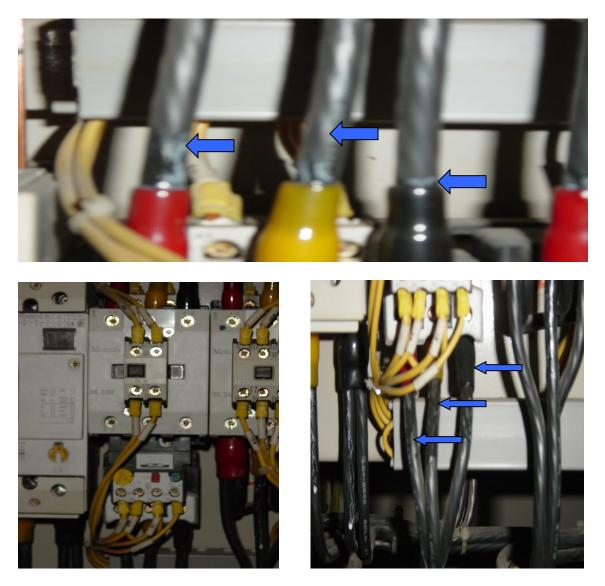
Deformation and discolourisation of cables are resultants of excessive heat loss from the cables and it might just weaken the whole cable insulation.
