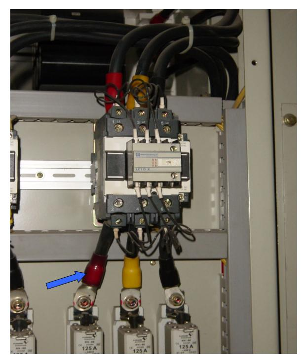
Carbonization on cable (might deteriorate the insulation and lead to flash over)
