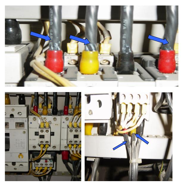
Insulation to the cables is deformed. Burn marks are found on both the cable and cable terminations.
