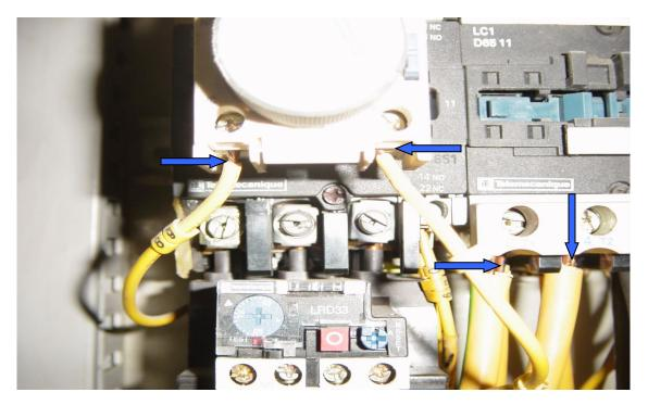
Burnt marks are found on the R phase (unbalance loading at load side). Measure the load at each phase (R, Y, and B) and try to balance or transfer the loading on each phase.
