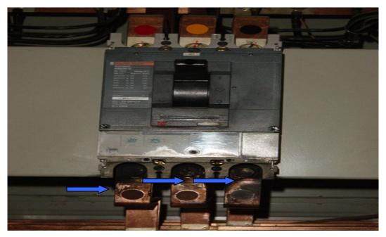
Burn marks on bus bar (clean and check for loose connections on bus bar during electrical maintenance).
