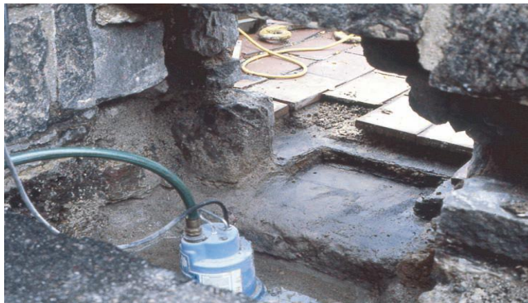
Figure 7: Exposing membrane for repair
