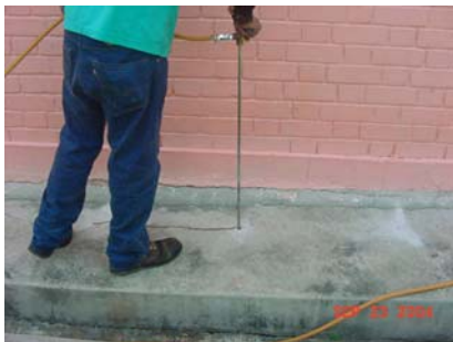
Chemical injection into the apron ground (soil) through the pre-drilled holes.
