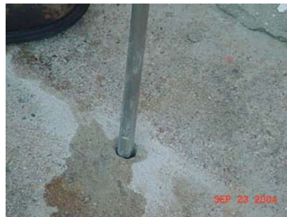
Chemical injection into the apron ground (soil) through the pre-drilled holes.
