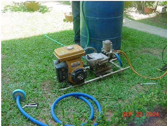
Pump used for the injection of chemical into pre-drilled holes.
