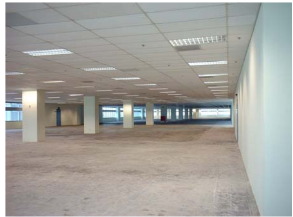
Overview of 5 th Level Unit
