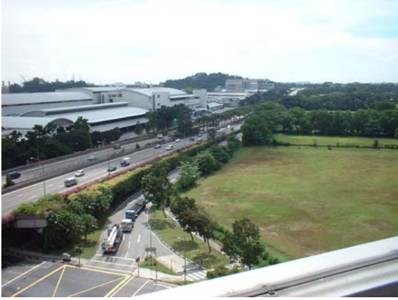
Building “C” – Southern Facing Expressway
