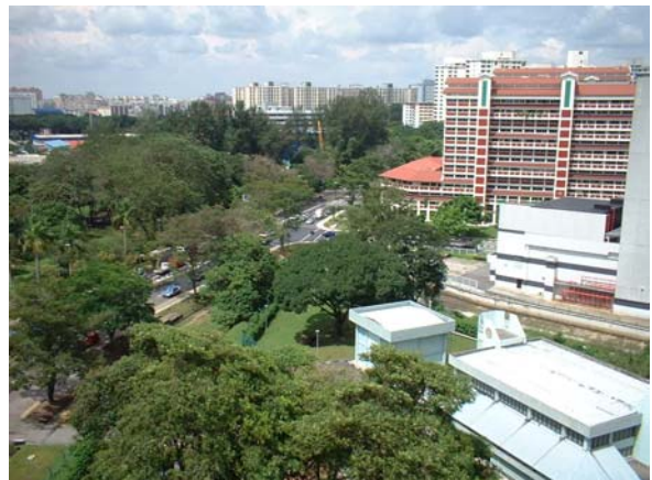
Building “C” – Northern Facing
