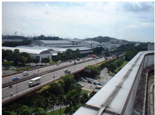
Building "C" – Southern Facing Expressway
