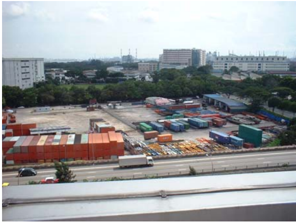
Building “C” – Southern Facing
