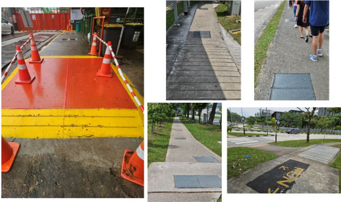
Figure 1 Some common coatings and features such as tactile and steel covering on pavements
